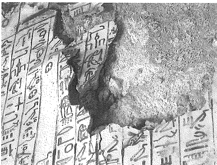
Figure 8. Detachment of stucco from the parent rock in the tomb-chapel of Djehuty. (See colour plate section, page 305).
